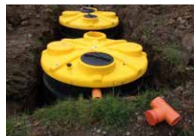
Domestic wastewater treatment (35 PE). Installation d'épuration eaux usées (35 EH).
