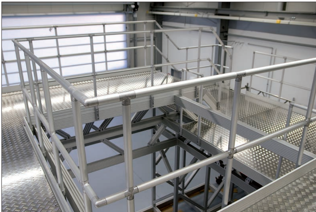
Working platform with ITAS railing
