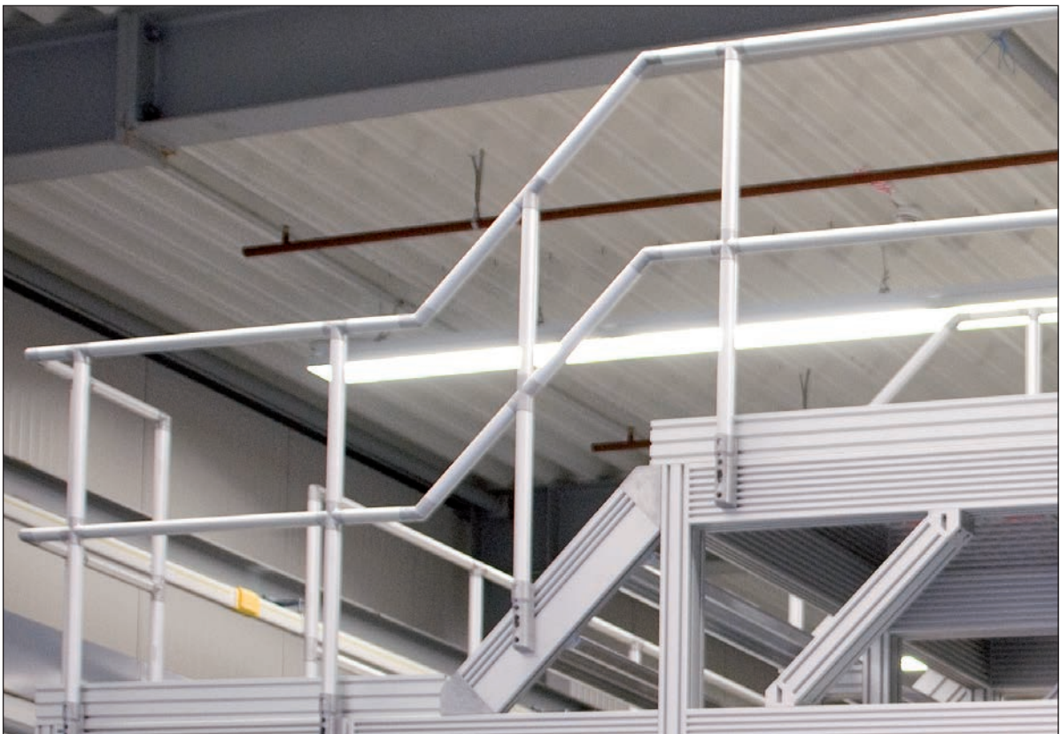
Staircase between two operating platforms.
