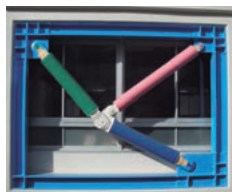
Toggle Type Vibration-proof Damper for Building Antiseismic Reinforcement
